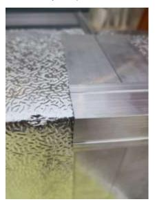
After the ventilation channels are connected, the cover cap can be placed around the corner to ensure a beautiful invisible finish of the connection. The corner cover cap can be fastened with sealant/glue onto the corners or with some self-drilling screws.
